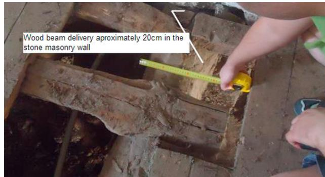
Fig. 4. Delivery of the wooden beam on the masonry wall (image adapted from: [9]).
