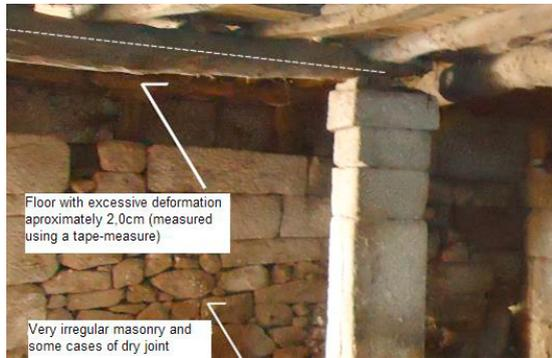
Fig. 2. Deformation of the beam under analysis (image adapted from: [9]).
