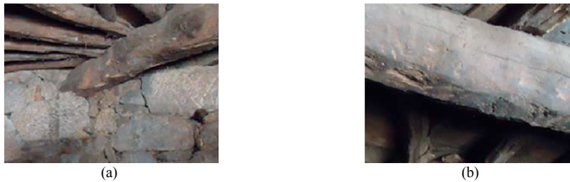
Fig. 5. Wooden beams supported by masonry walls (images from: [7]).
